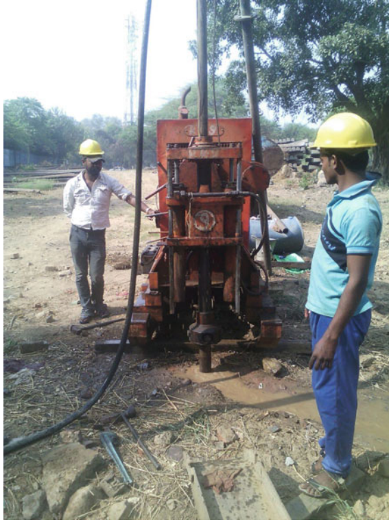
Fig. 18.2 Borehole drilling in progress
