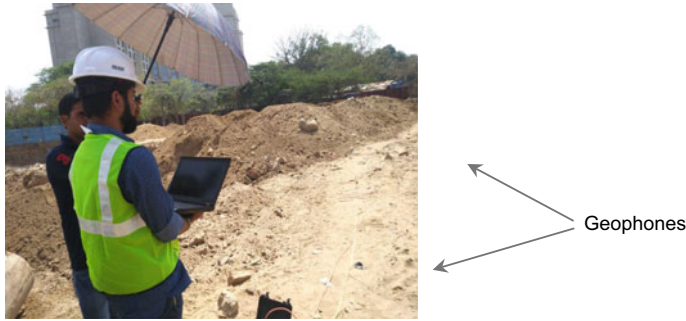
Fig. 18.4 Seismic refraction test—data acquisition in progress
